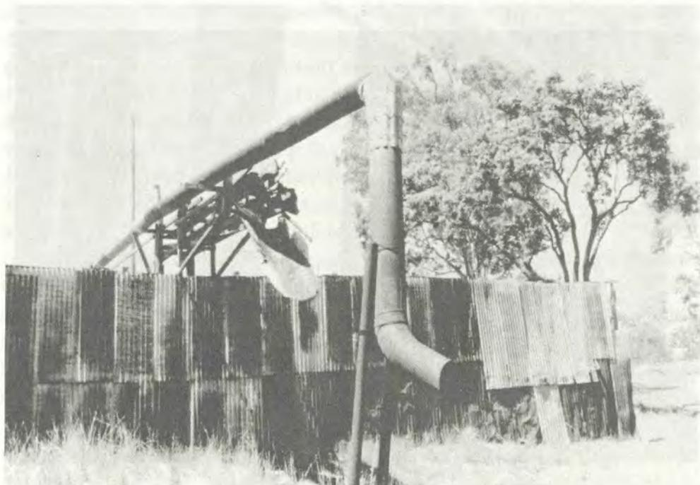
Burning area for waste sawdust and planing shavings. The corrugated iron fence was constructed to prevent sparks from the fire blowing back towards the mill where they would have created a fire danger. Photographed December 1995.
