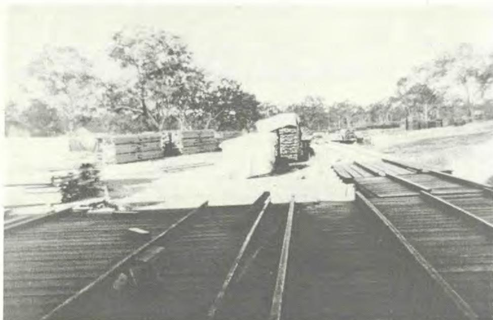
View of the timber yard on the eastern side of the mill, taken in 1982, showing the tram tracks. The trolley that can be seen on the right at the end of the mill was moveable, left or right to be aligned with the rails, each of which came from one of the saws. The trolley could then be pushed into alignment with the tracks that can be seen running into the timber yard.
