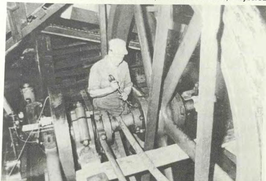
A new big end bearing and crankpin were fitted to the engine and the flywheel was checked on the crankshaft. January, 1984.
