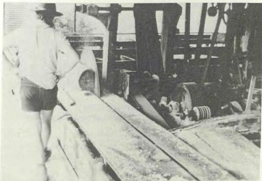
A small log going through the breaking down bench, only the bottom saw is in place for this log. January, 1986.
