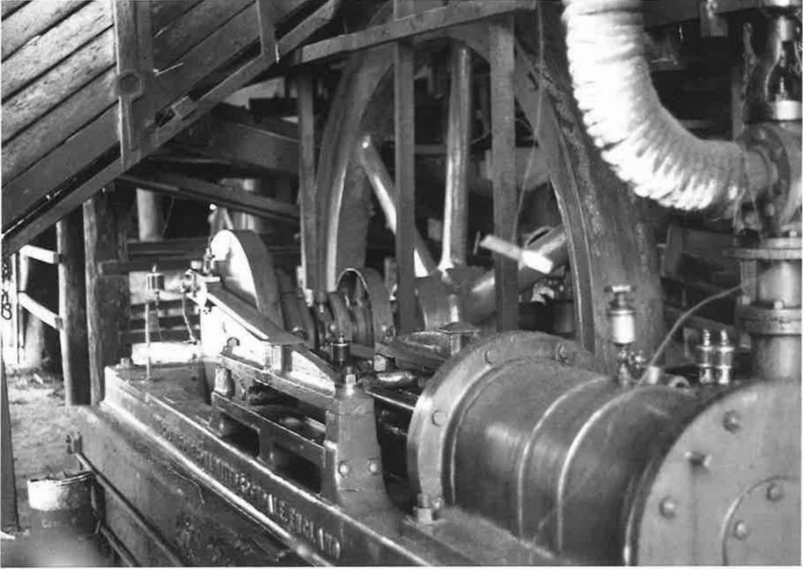
A view of the engine from the cylinder end. The wooden chute seen in the top left hand corner of the picture carried sawdust and wood scraps from the mill floor above to the front of the boiler furnace situated to the left.
