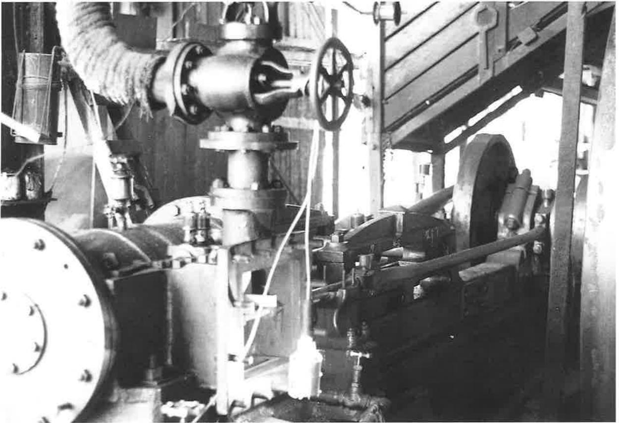
Photo shows the steam chest cover removed and the "skeleton valve" in position resting on the valve spindle. The lead light hanging down from the throttle valve spindle was plugged into a nearby power point, one of only a few in the mill. These together with a few lights were the only mains electricity supply available.
