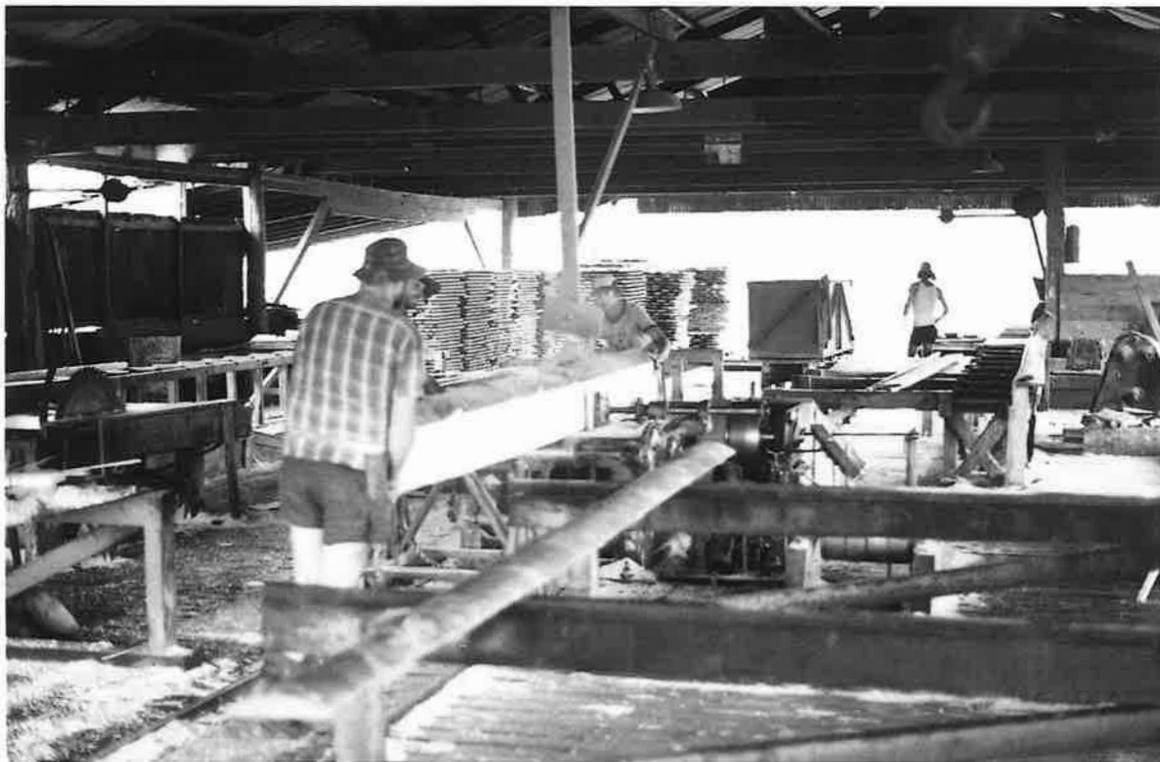
A large slab of pine is being handled by a man at each end of the heavy No. 1 saw bench, while a third man, nearly obscured by the man closest to the camera, controls the cut with the simple reversible three cylinder radial steam "feed" engine.
