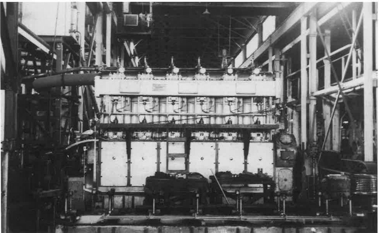
Photos opposite depict a 550 HP "E Class" freighter engine on the test bed prior to being transported down to the Kent St. Shipyards and lowered into the new hull using the sheer legs crane.
