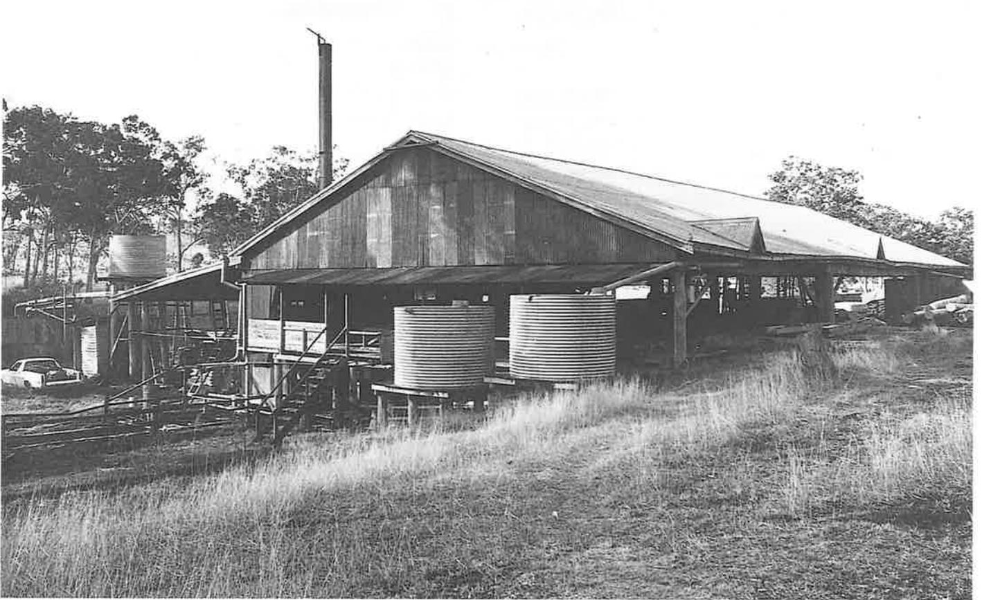
The mill was built on a slope running down to the creek which supplied the boiler feed water. This was pumped up into the high tank on the left. The two tanks on the right held rainwater caught off the roof.
