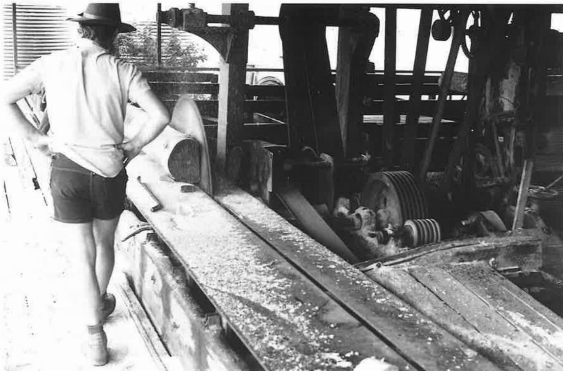
A skilled operator walks alongside the moving table or bench as the cut finishes and the flitch falls to the rails seen in the background, for transfer to the Number 1 bench. The Canadian was often referred to as a Rack bench, due to the fact that it is driven through a long gear rack fixed to the underside of the table.
