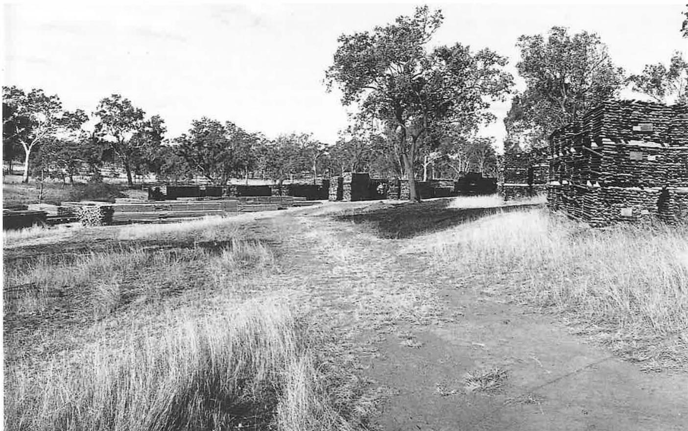
The large open spaces at the far end of the mill held many big stacks of pine planks carefully stripped up for natural air drying. All were cut with power supplied by the old Robinson engine.
