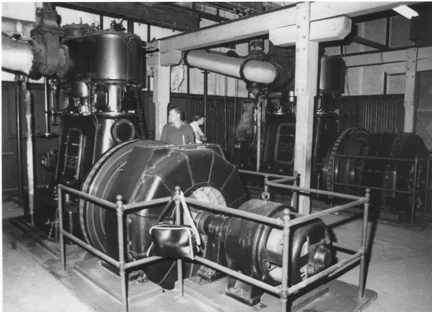
Wilson Hart & Co. Engine Room showing the two Belliss & Morcom Steam Generating Sets installed after the 1934 fire.
