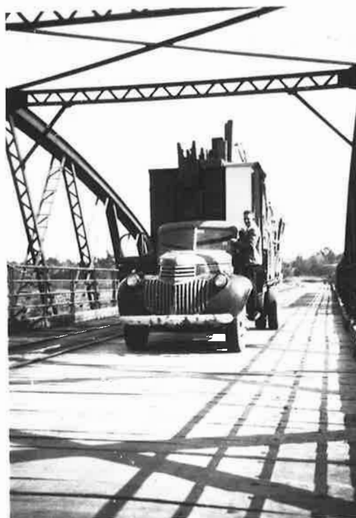
Bulmer's truck on bridge prior to curbing.
