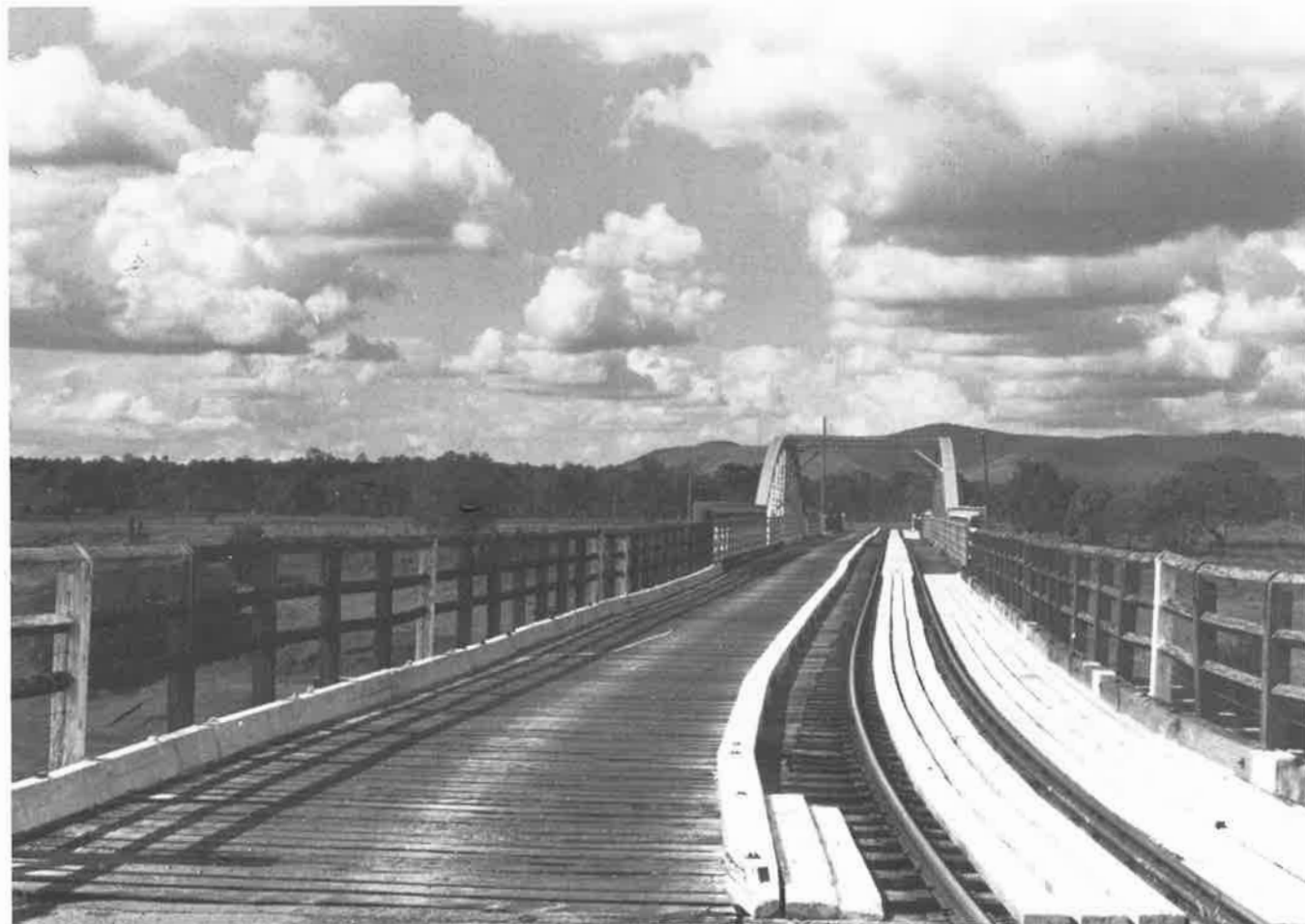
Bridge showing curbing.
