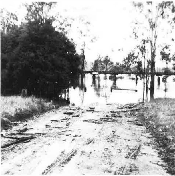
Flood at Sawmill Bridge.
