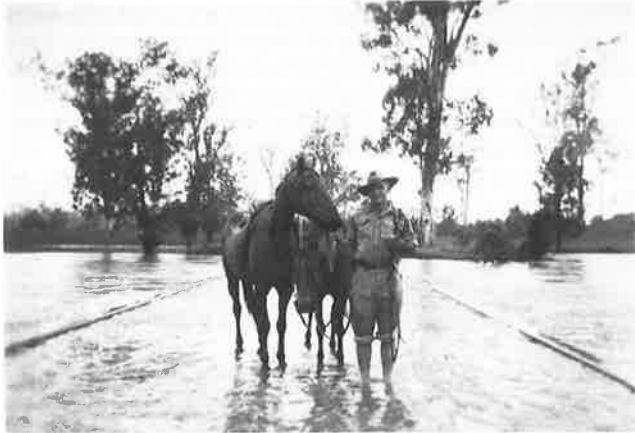
Miva Crossing Bridge
