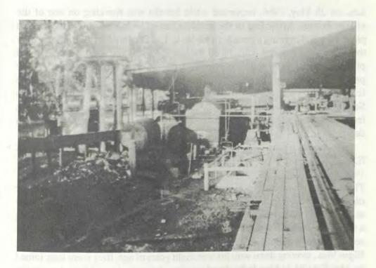
Western side of the mill showing boilers and engine. Note the pier and tracks leading to rubbish tip. This is where William Otto Schultz was killed.
