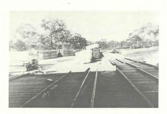
View of the timber yard on the eastern side of the mill, taken in 1982, showing the tram tracks. The trolley that can be seen on the right at the end of the mill was moveable, left or right to be aligned with the rails, each of which came from one of the saws. The trolley could then be pushed into alignment with the tracks that can be seen running into the timber yard. Source—Peter Olds, Wm. Olds and Sons, Maryborough
