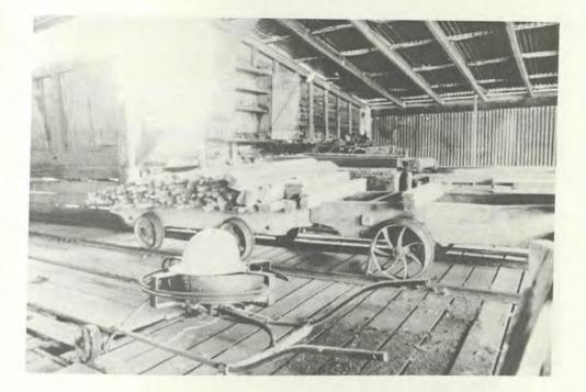
Timber trolleys such as this ran from each of the benches to another larger trolley running along the eastern side of the mill. This larger trolley could be aligned with all the tracks running from the saw benches and then aligned with the rail line running through the timber stacking yard. In the background of this photograph is the area that once accommodated the planing machine. Photographed December 1995.
