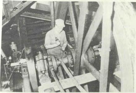
A new big end bearing and crankpin were fitted to the engine and the flywheel was checked on the crankshaft. January, 1984. Source—Peter Olds, Wm. Olds and Sons, Maryborough
