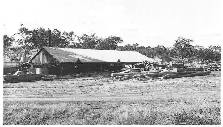
Timber trucks dumped their log loads on the top side of the mill where they were easily loaded on to the moving carriage of the Canadian Bench for breaking down.
