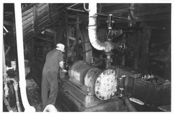
Reassembly has been completed and the Piston Rod Gland is being repacked prior to a test run.
