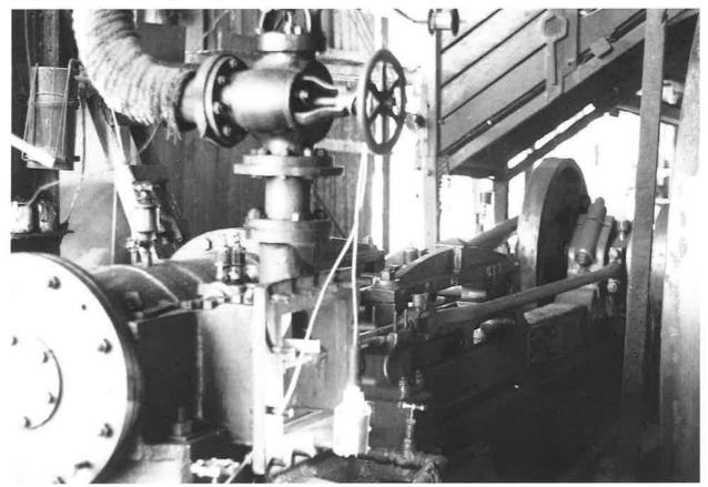
Photo shows the steam chest cover removed and the "skeleton valve" in position resting on the valve spindle. The lead light hanging down from the throttle valve spindle was plugged into a nearby power point, one of only a few in the mill. These together with a few lights were the only mains electricity supply available.
