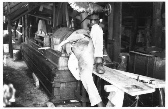
The bore, steam ports and steam chest are throughly cleaned out prior to assembly.
