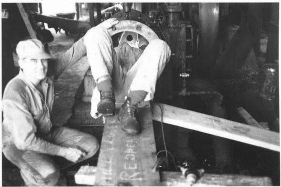
The cylinder bore was ground out and scraped to remove ridges or steps in the bore at the ends of the stroke of the old piston. Leading hand fitter machinist Alan Johnston is at the left, with third year apprentice fitter machinist John Petersen lying in the bore of the 16 3/8 inch diameter cylinder.
