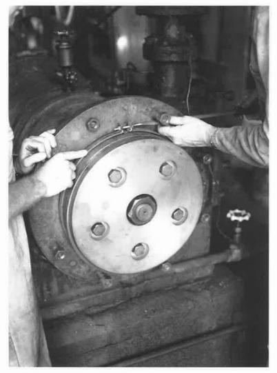
The piston has been entered into the bore and the piston rings are being compressed in order to get them started into the bore also.
