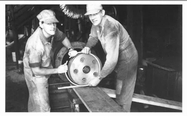
The new piston rings were first checked for "gap clearance" in the bore and then fitted to the piston. John Petersen at left with Alan Johnston.
