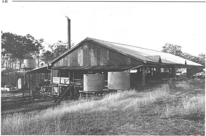
The mill was built on a slope running down to the creek which supplied the boiler feed water. This was pumped up into the high tank on the left. The two tanks on the right held rainwater caught off the roof.
