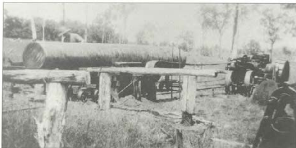
Breaking-down saw at Charles Baldwin's sawmill on his property at Oakview.
