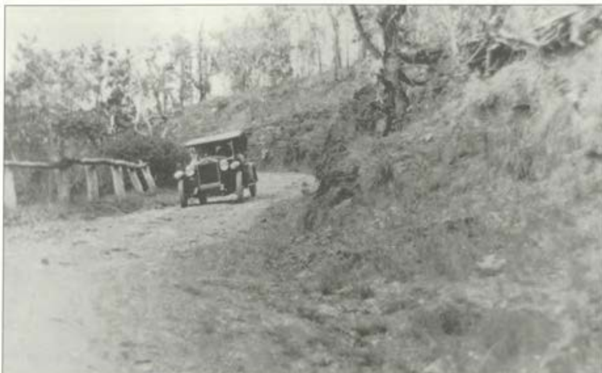
Les Wieden's mail car travelling up the Blackbutt range. This form of transportation was vital to residents in rural areas such as the South Burnett, providing communication and transport facilities to the cities. The cars were licensed through the local government authorities.
