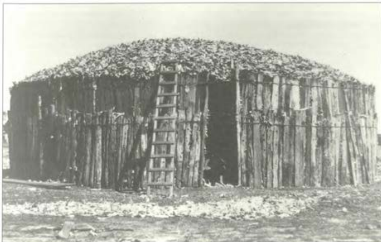
Unusual type of circular corn crib in use on J. Petersen's farm at Home Creek, photographed 23 September, 1934. It had a circumference of 45 yards, 10 ft. wall with crown 4 ft. higher, giving a capacity of about 1300 bags. It was loaded with nets and a crane from a wagon; unloading was done from a self-feeding passage. One man fed 660 bags in 1½ days.
