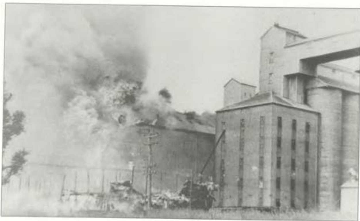
Kingaroy peanut silo fire, February 1951.
