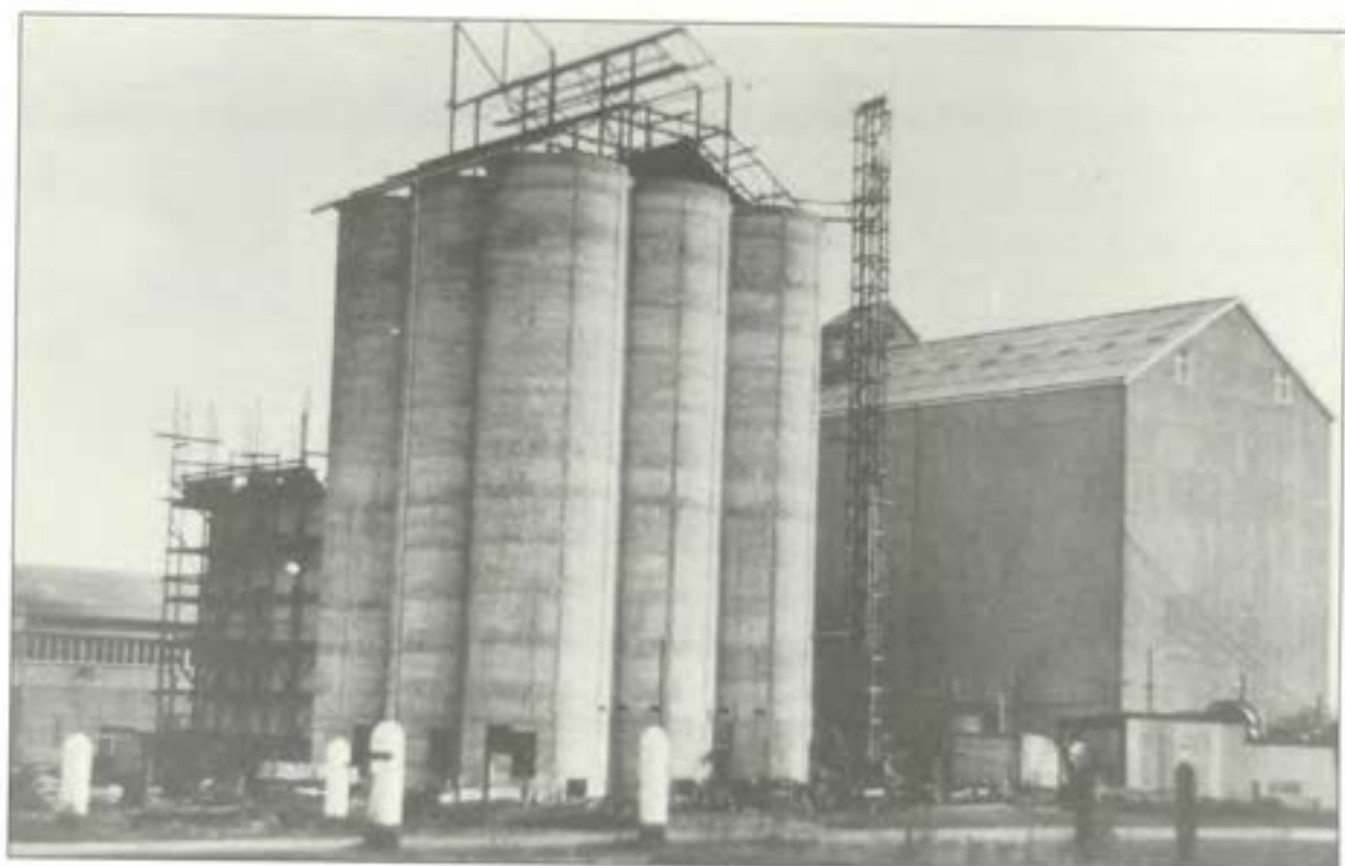
In 1938 the second group of silos were constructed at a cost of £57,750.
