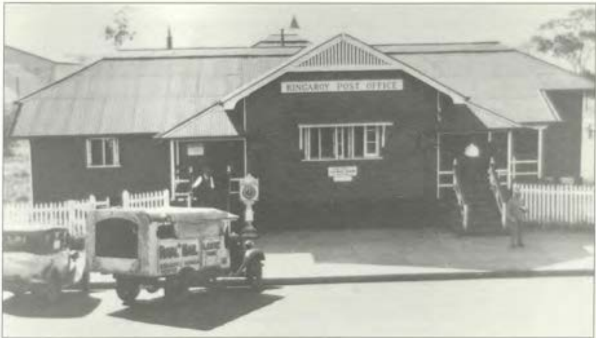
Kingaroy's first post office, erected in 1907, on land donated by Arthur Youngman, on the corner of Kingaroy and Alford Streets. The photograph depicts the building with extensions and improvements as it was on 21 March, 1935. It was replaced by a new post office on the same site, opened on 31 March, 1958. The town's first telephone exchange was opened on 4 October, 1911; this was a manual switchboard with 32 subscribers' services. On 8 December, 1953, magneto type telephone exchange equipment was replaced by common battery equipment. 785 subscribers' services were transferred to the new exchange.
