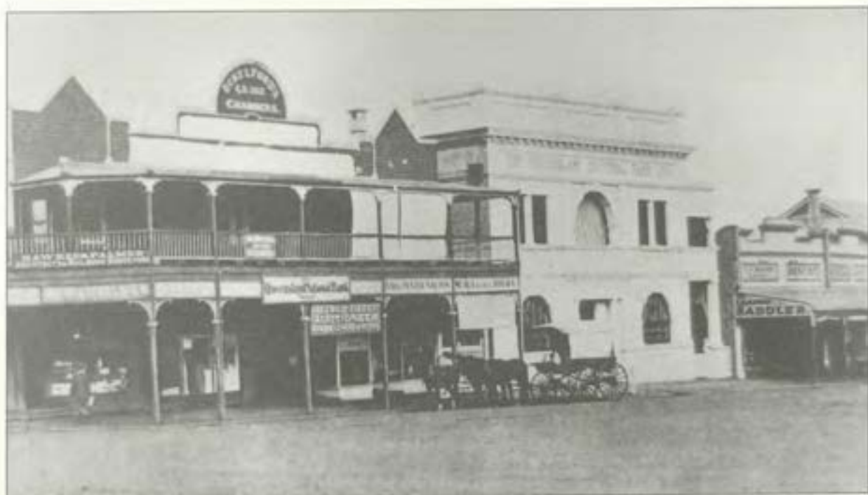
In 1912 Ockellford's Chambers were completed by adding a second floor over the existing shops. Neilsen's saddlery shop was removed to Haly Street and Staines Brothers' shop was pulled down to make way for the Q.N. Bank erected in 1914.
