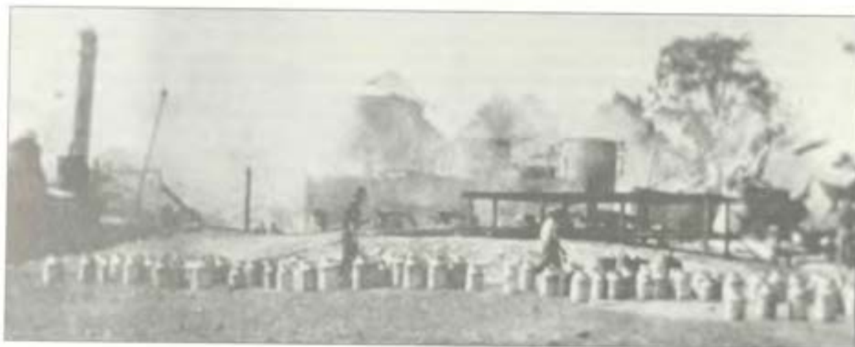
The second factory fire at Nanango, 13 October, 1926.
