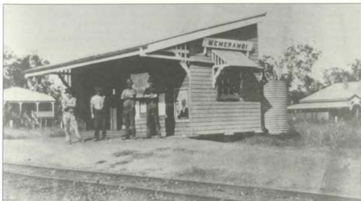
Memerambi railway station. The extension of the railway from Wondai to Kingaroy gave Memerambi its rail connection when the line was opened on 19 December, 1904. Source — Kingaroy Shire Council, Harold Mears' collection.
