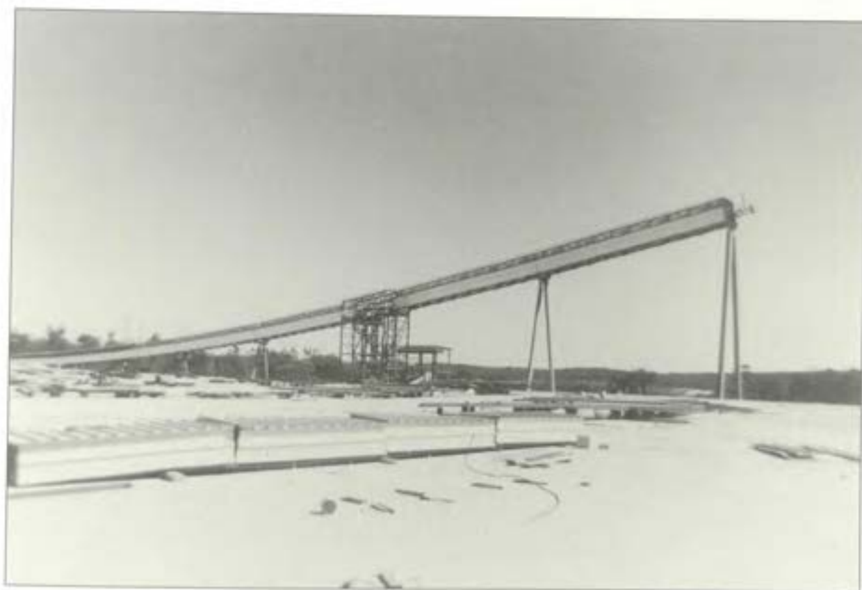
R1 conveyor from Pacific Coal's product load-out bin showing drive and take-up tower, 9 May, 1983.
