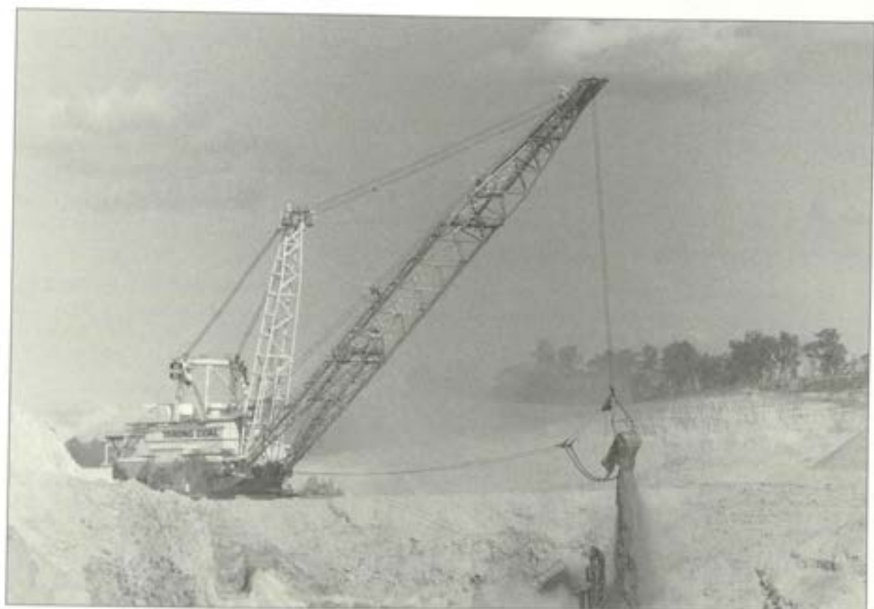
The drag line at Meandu mine clearing overburden.
