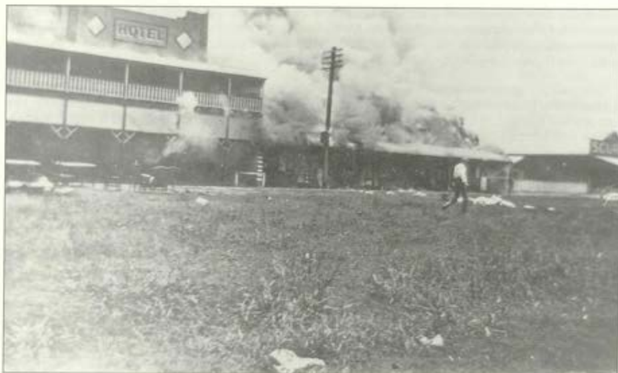
Destruction of the Royal Hotel at Murgon, 16 January, 1928.
