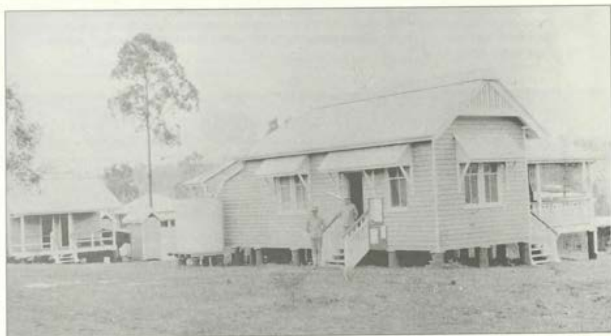
Police station, Blackbutt, 1914.
