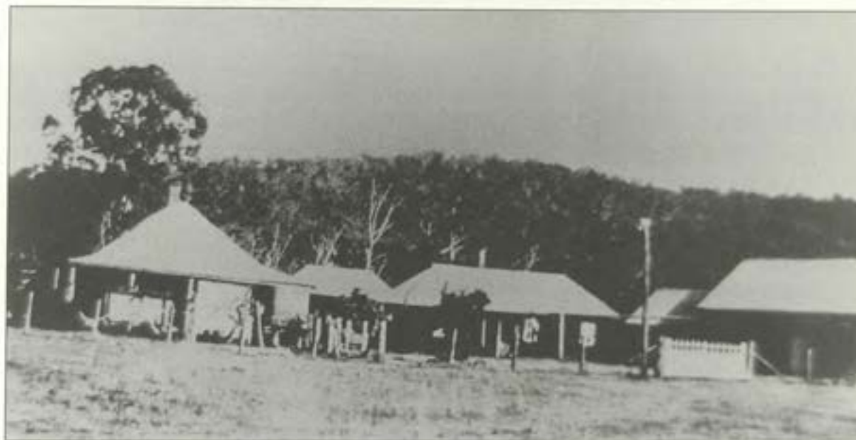
The original Taromeo station homestead, later destroyed by fire.
