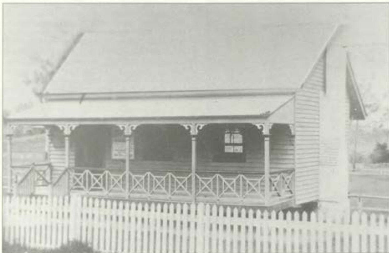
Original shire office, Kilkivan, 1914.
