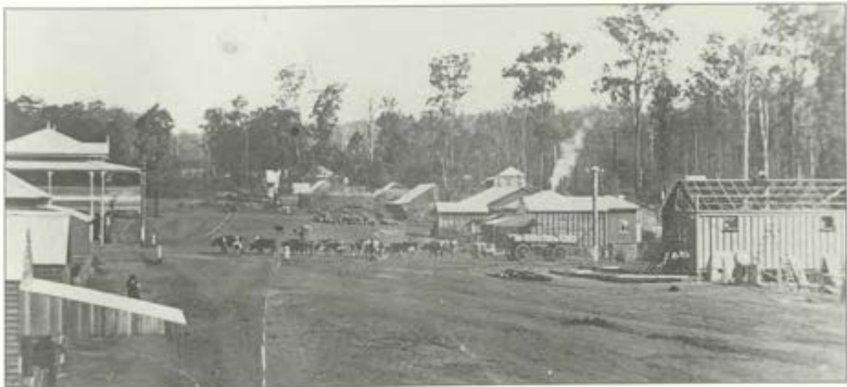
The developing township of Blackbutt, 1900s.
