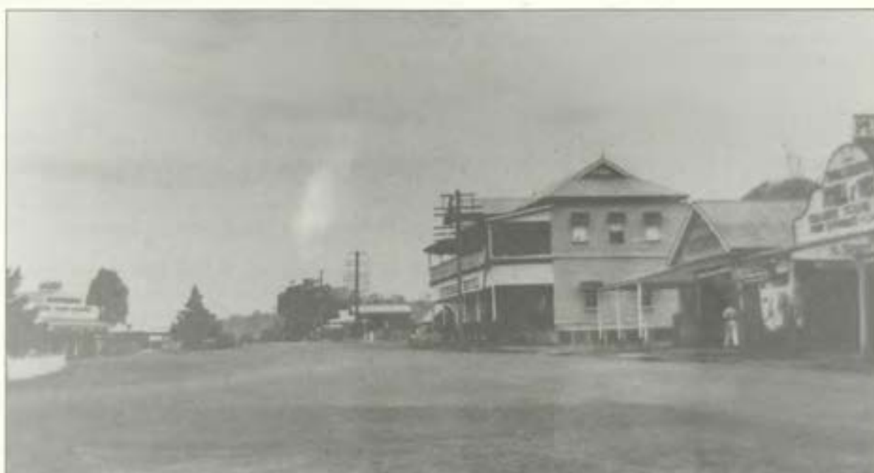
Bligh Street, Kilkivan, looking east.
