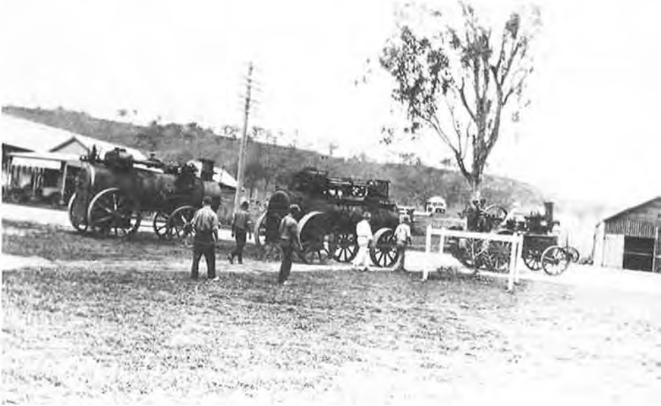
Compressors for Cinnabar Quicksilver Mine leaving Kilkivan
