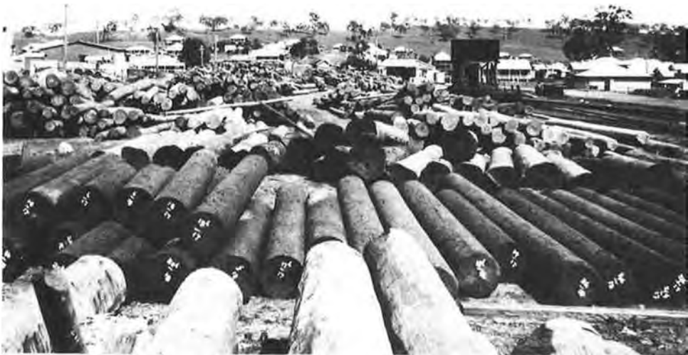
Timber yard at Goomeri Railway Station
