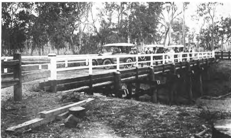
Opening the Bridge at Tansey
