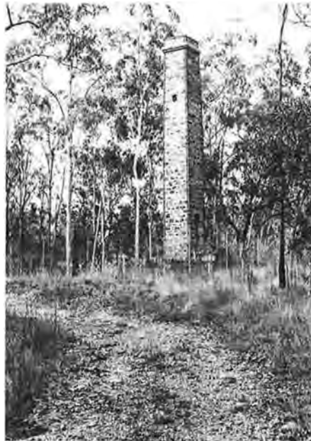
Mt Clara Copper Smelter Chimney
