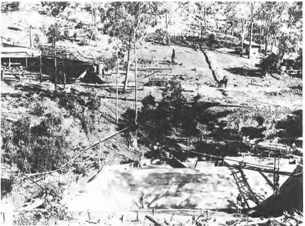
Water Storage Dams - Mudlo Mine
