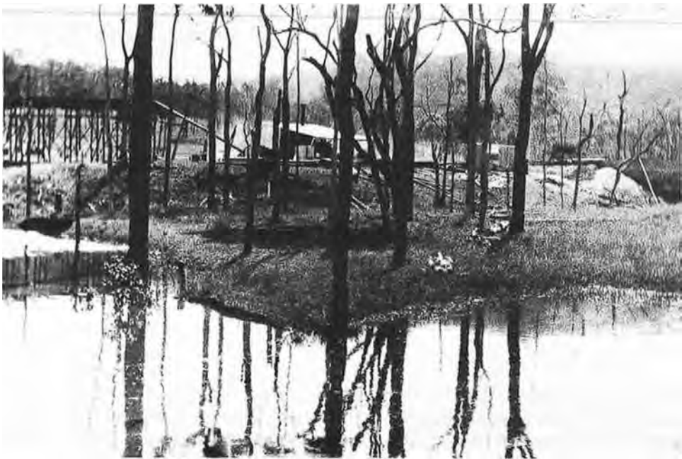
Cinnabar Quicksilver Mine - water storage dam (Kilkivan Historical Society)
