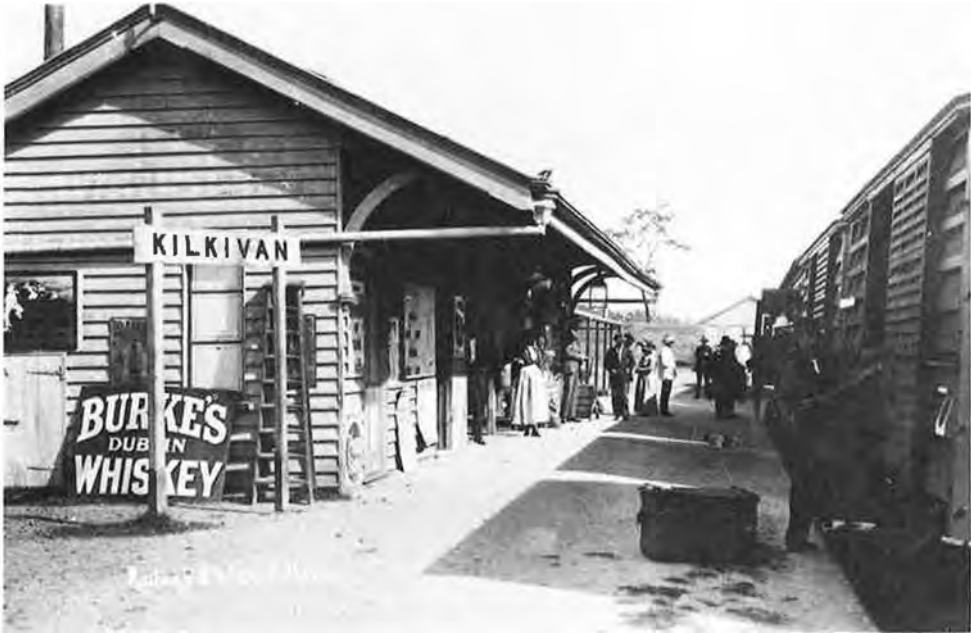
Kilkivan Railway Station - 1911
