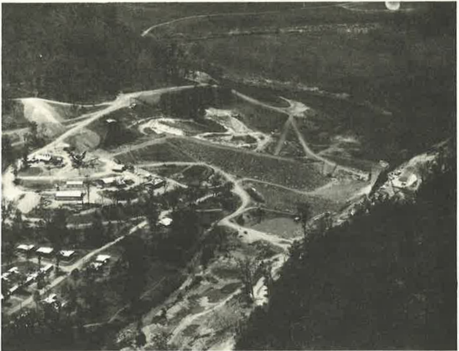
Aerial view of Borumba Dam during construction
