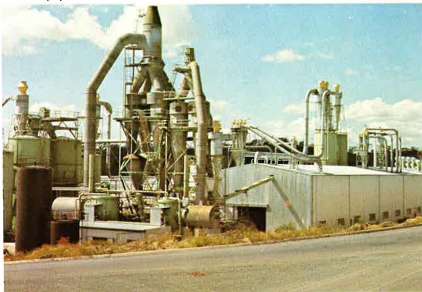
'oodland Ltd.'s big board manufacturing plant on the southern outskirts of Gympie.
