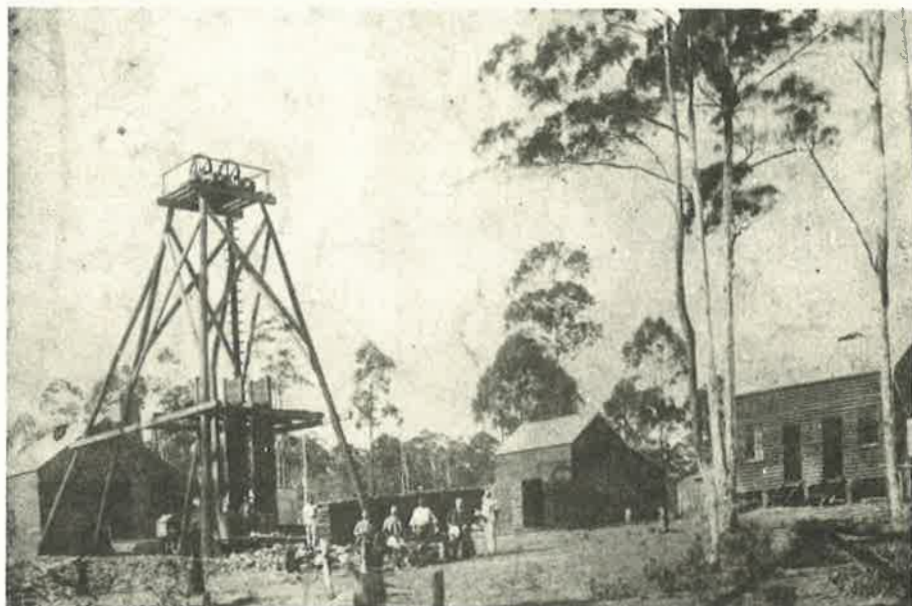
Headworks at the Enterprise mine
