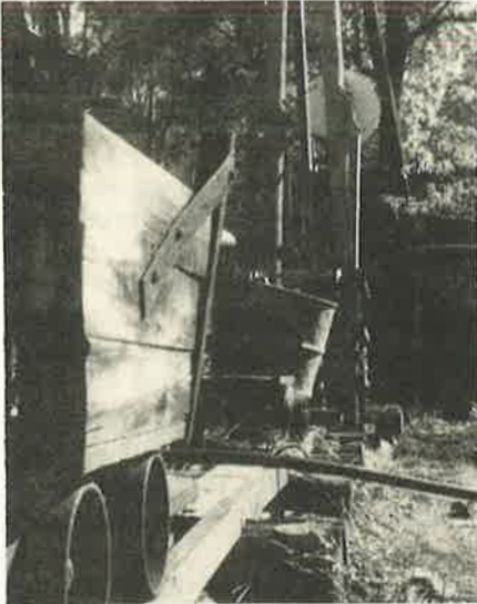
Headworks at Neerdie mine
