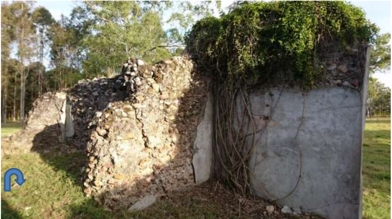
Remains of Hugo's dairy at 95 Stumm Road Gympie-blue marks a drainage hole from the dairy. Note the thick walls of the dairy which were originally rendered with concrete
