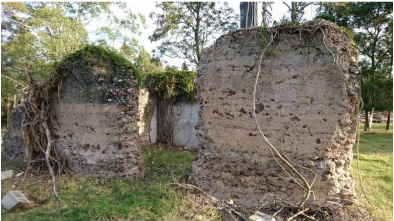
Remains of Hugo's dairy at 95 Stumm Road Gympie-blue marks a drainage hole from the dairy. Note the thick walls of the dairy which were originally rendered with concrete
