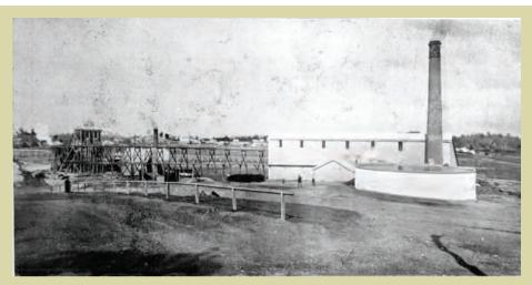
Mine buildings including tramway, battery and concrete water tank at the eastern shaft of the 2 South Great Eastern in 1903. Today the tank is part of the display area of the museum. Source: The Gympie Times, 1903.
