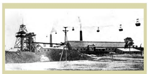
In 1911, a flying-fox (aerial tramway) was constructed to deliver ore from the No.3 shaft (unseen on right) to the crushing battery adjacent to the No.1 shaft. Source: (Keith Waser Collection) Gympie Regional Libraries.
