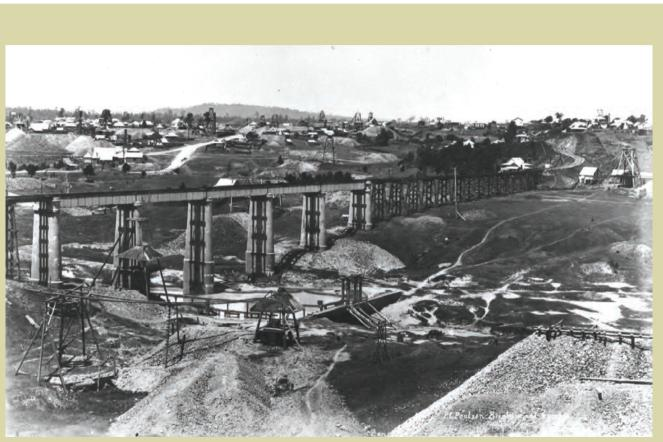
The Deep Creek bridge on the Brisbane rail line, circa 1899. Note mullock, old shallow shafts and weir in the foreground and numerous headframes at Monkland in background. On the left above rail bridge is the Victoria battery. Photographer: P. Poulsen. Source: Lees, W. 1899.
