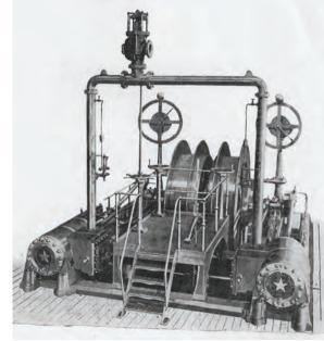
A steam winding engine manufactured by Walkers Ltd for the Oriental Consols Gold Mining Company in 1900. This plant consisted of a pair of coupled twenty inch cylinders with forty-two inch stroke and a pair of eight foot drums with a one inch rope 2,750 feet in length. The Cornish boiler was twenty-seven feet long and seven feet in diameter. Source: The Gympie Times, 1910.
