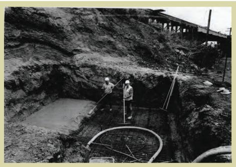
The Shaft Capping Project team places a concrete cap over an exposed mineshaft. Source: The Gympie Times.
