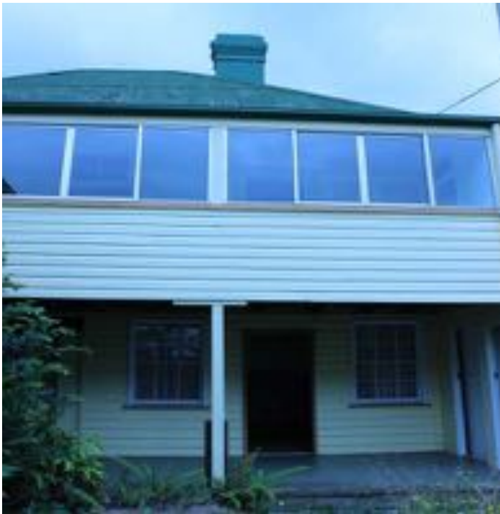
View of the rear of 34 O'Connell Street
