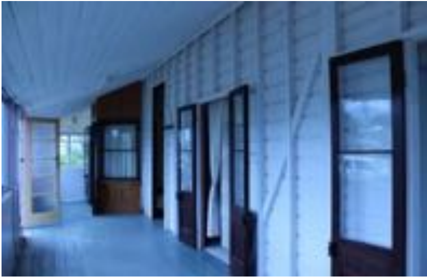
View of the inside closed in verandah coming in from the front entrance of 34 O'Connell Street Gympie
