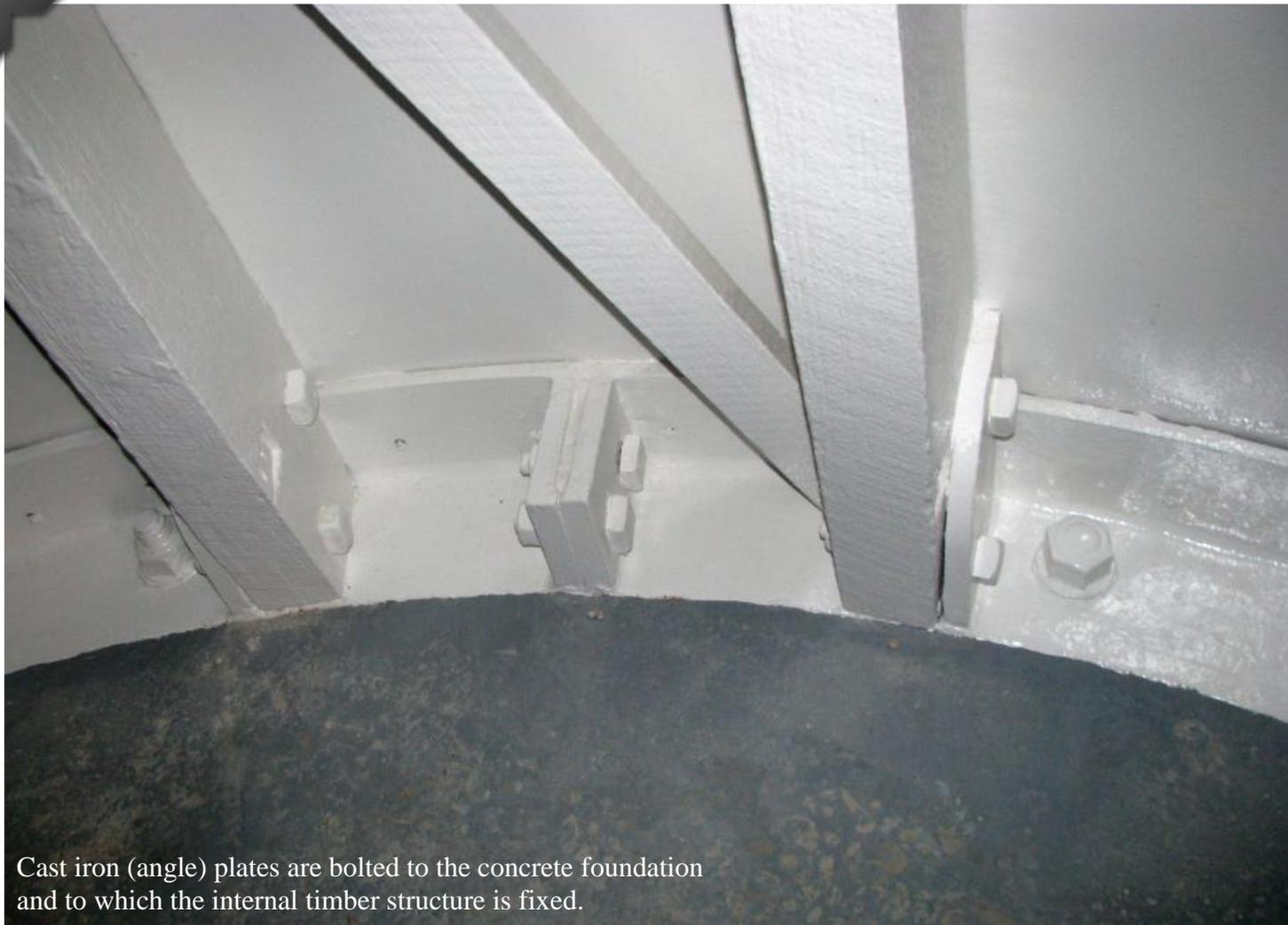
Cast iron (angle) plates are bolted to the concrete foundation and to which the internal timber structure is fixed.
