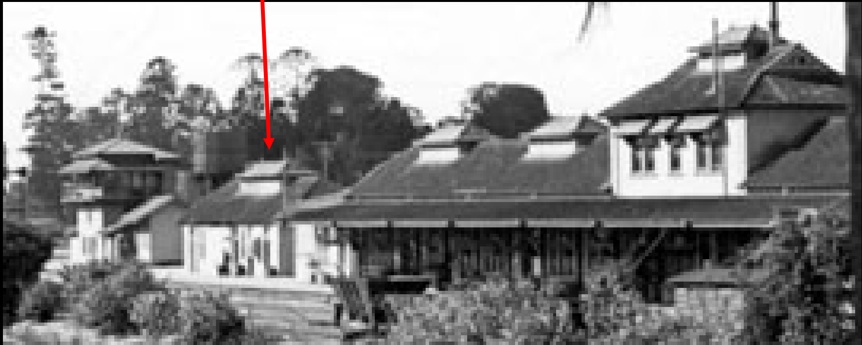
Building housing Lamp/porter/guards room with pagoda roof c1940 Picture Sunshine Coast
