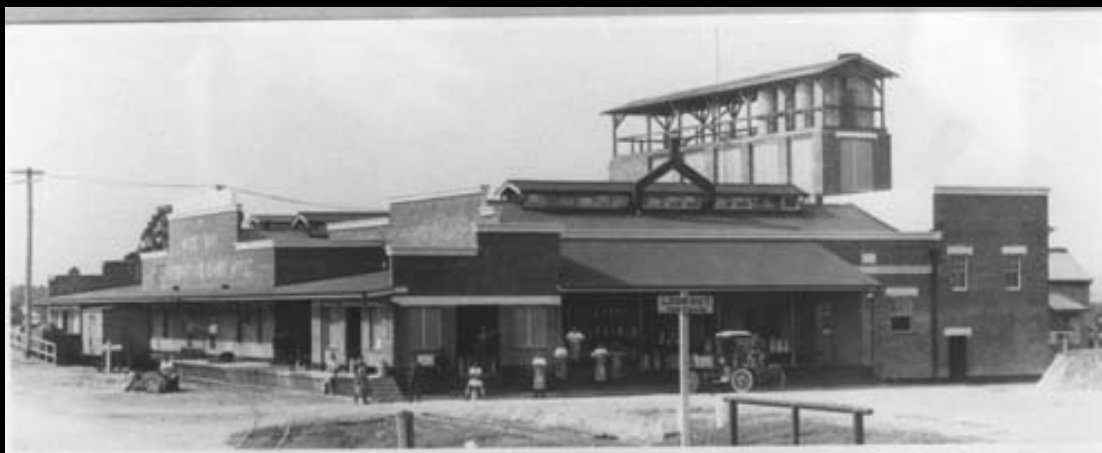
BUTTER FACTORY—Designed and Built by Messrs. J. Wildridge & Sinclair (Brisbane), Ltd., Australia, for the Wide Bay Co-operative Dairy Association Ltd., Gympie.
