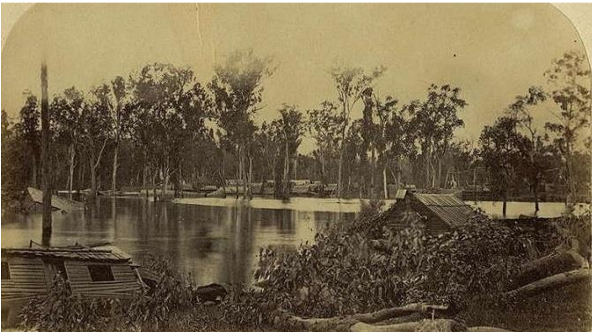
Timber houses submerged in the Gympie floods, 1870 19
