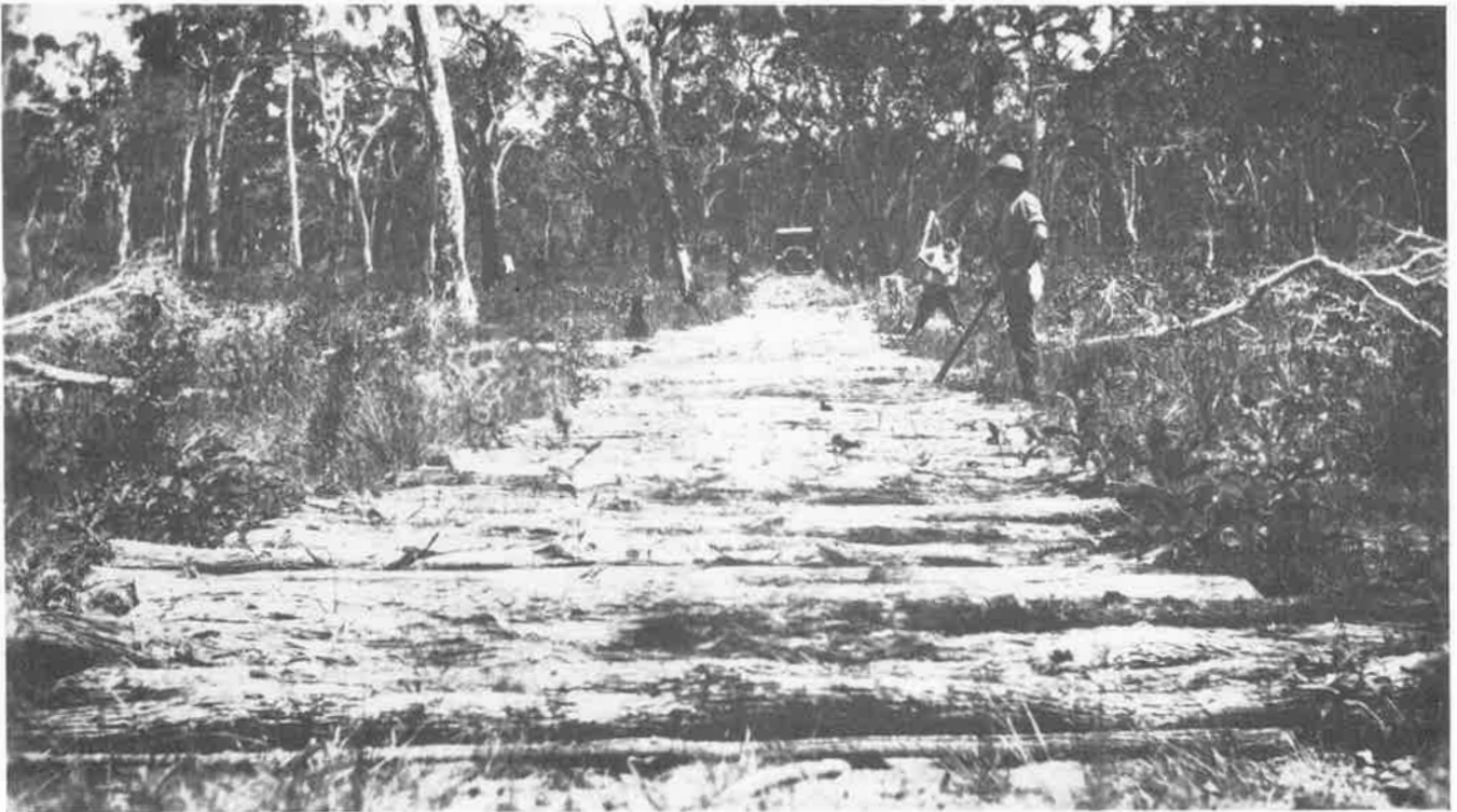
Building a road over a wet boggy patch. This was called "corduroy". Sections of log were placed side by side.
